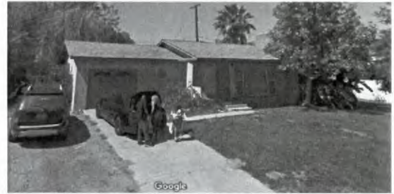
13 After IH installed a new roof (no permits issued):
