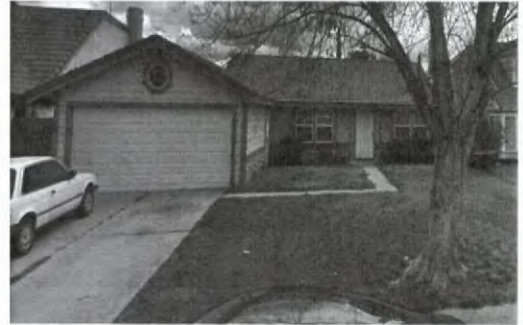
After Solar Panel Removed (no permits issued):
