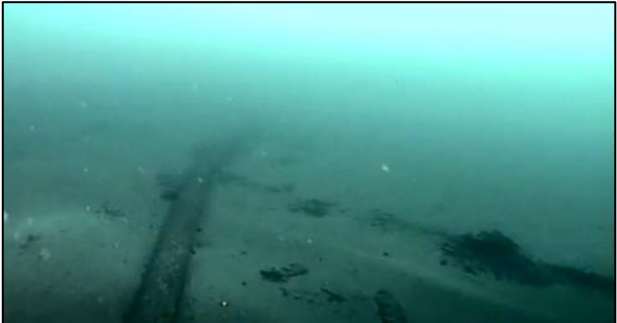
27 28 Image 7, Movement of Pipeline
